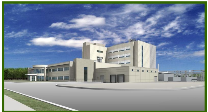
Figure 1.2: Isometric View. (Courtesy of Project Architect) The Production Building is the five-story building in the back.
